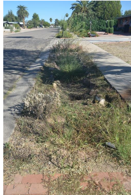
Curb-adjacent stormwater collection basin, 5500 block of East Alta Vista, Tucson, AZ, Oct. 26 (Photo by: Denise Meeks, 2021).
