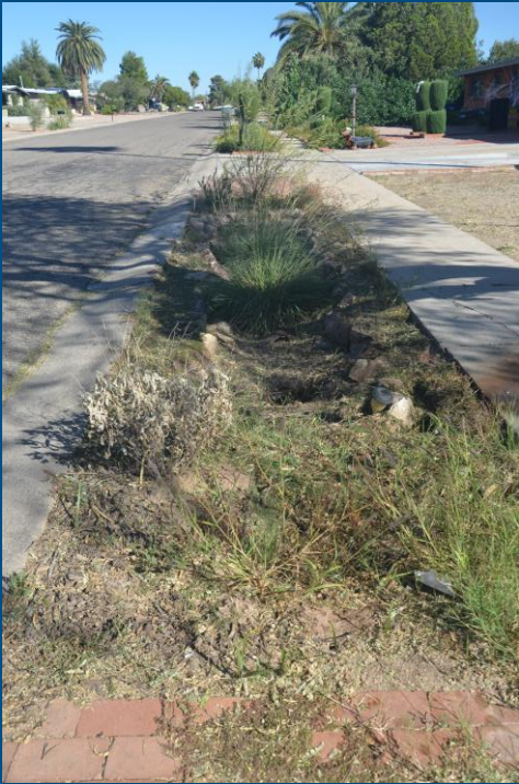
Curb-adjacent stormwater collection basin 5500 block of East Alta Vista Green Stormwater Infrastructure Grant Project D. Meeks Oct. 26, 2021 Image taken by and used with permission of the author CC BY-SA 4.0
