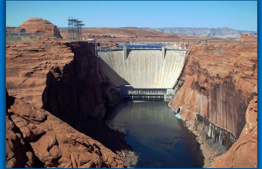
Glen Canyon Dam, substation and bridge near Page, Arizona Adbar Mar. 1, 2010 Wikipedia Glen Canyon Dam https://en.wikipedia.org/wiki/Glen_Canyon_Dam#/media/File:Glen_Canyon_Dam_and_Bridge.JPG CC BY-SA 3.0
